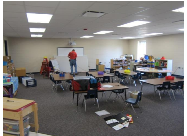
Findorff's carpenters installed the final white boards on Friday.
