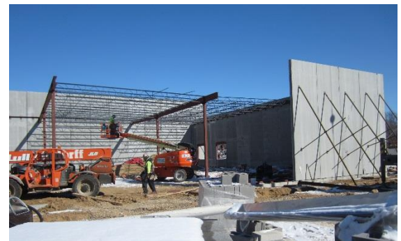
Ironworkers set roof joists for the new GTT area.
