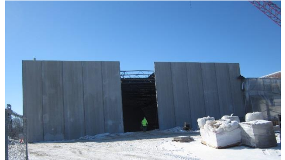
The new gym is nearly fully enclosed.
