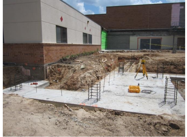
Footings are in place for the new 5 th grade wing.
