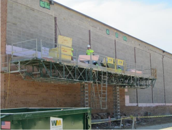
Masons remove the brick from the existing gym. The gym will remain and a new wall will be built next to it.
