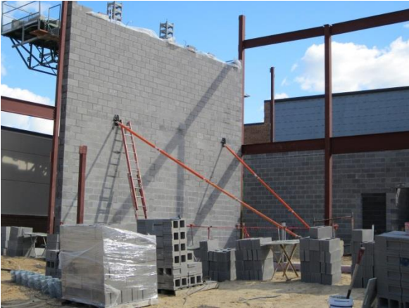
Temporary bracing is placed on the masonry walls in the 5 th grade wing to secure them until rest of the structure is complete.
