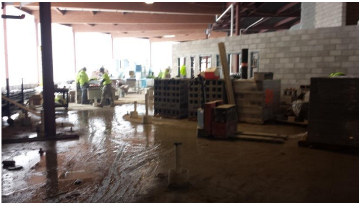
Inside the cafeteria, masons are laying block for the interior walls.
