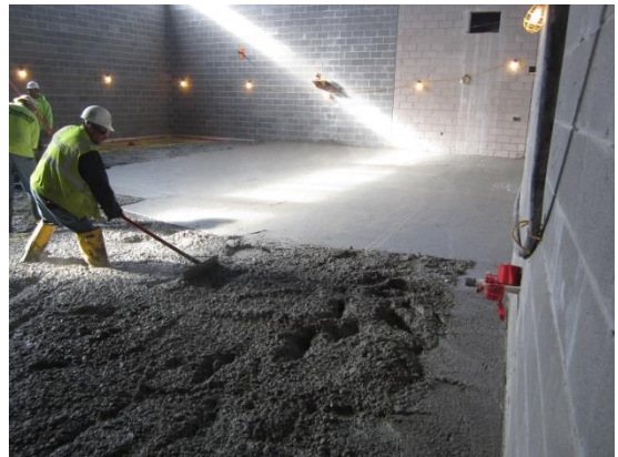
Workers place concrete in the new band room.
