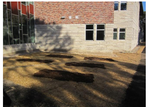
The school gardens have been created on the southwest end of the building – site
