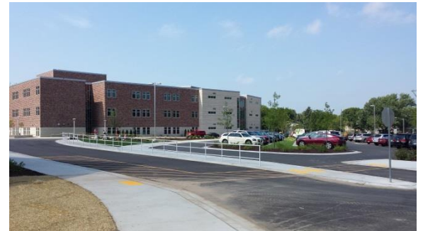
Landscaping is complete in front of the school– Site
