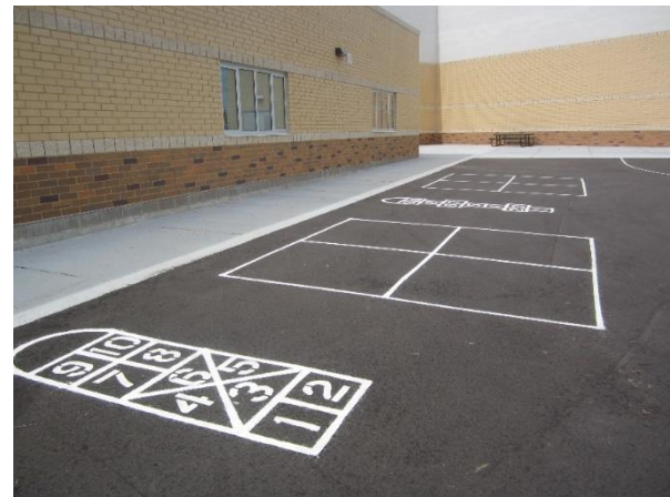
Asphalt top coat and striping are complete on entire site - Site
