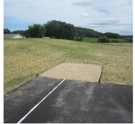
Long jump sand pit has been installed for track - Site
