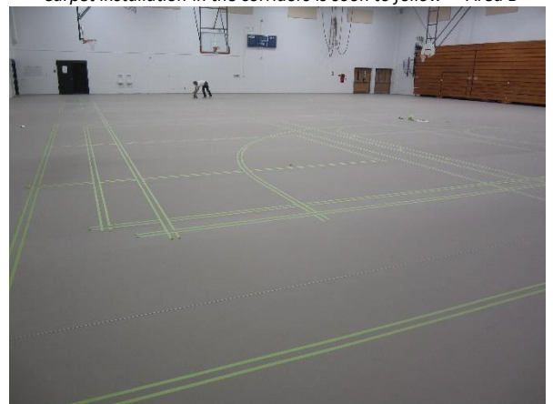
The synthetic gym floor is being striped with court markings – Area D
