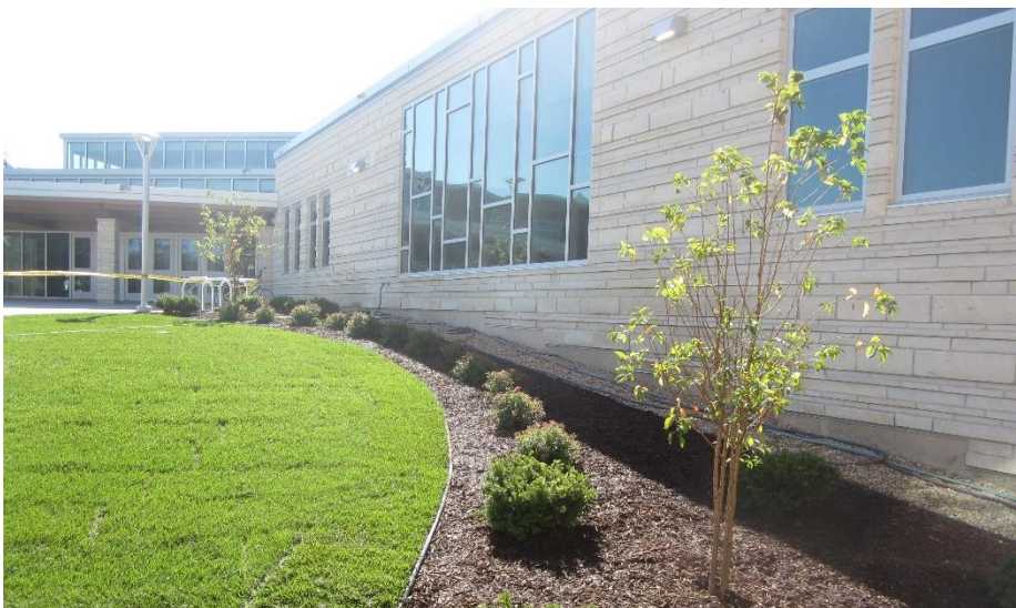
Sod and plantings are in place near the main entrance - Site
