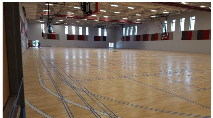
Gym floor striping is laid out and being painted!
