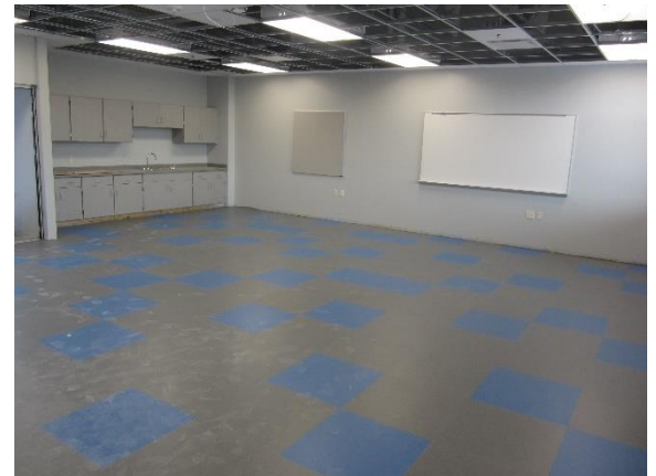
Vinyl floors and marker boards have been installed in the eastern 8 th grade classrooms – Area B
