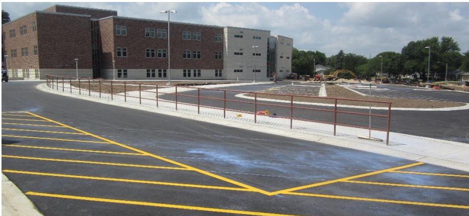
The main parking lot has been paved and striped - Site
