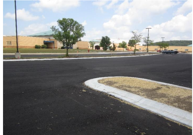
Asphalt binder course in the main parking lot is complete - Site
