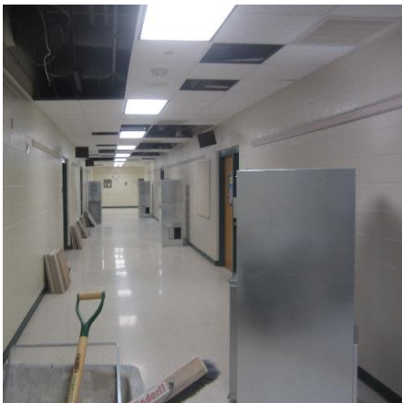
Old heat pumps have been removed, and new heat pumps are ready to be installed. – Existing building
