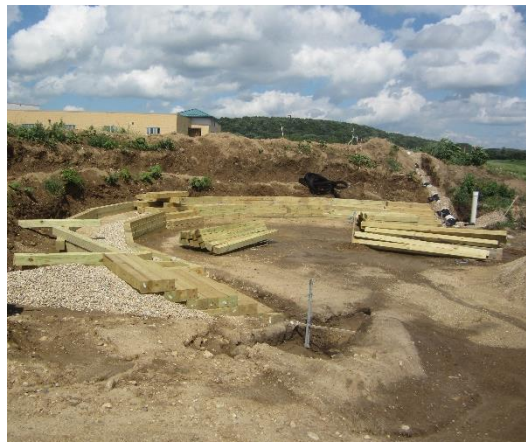
Seat walls for the amphitheater are being installed - Site
