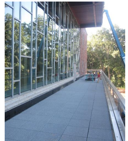
Roof pavers are in place on the library patio – Area B
