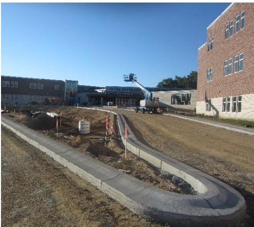
Concrete curb has been poured in the main parking lot and at the receiving area - Site
