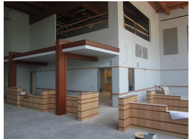
Installation of casework in the library is ongoing – Area B
