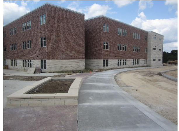
Sidewalks are being poured at the bus drop-off area - Site
