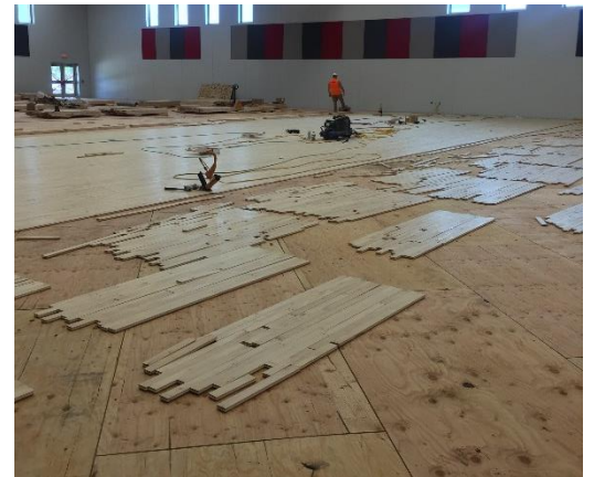
Wood flooring is being installed in the gym.
