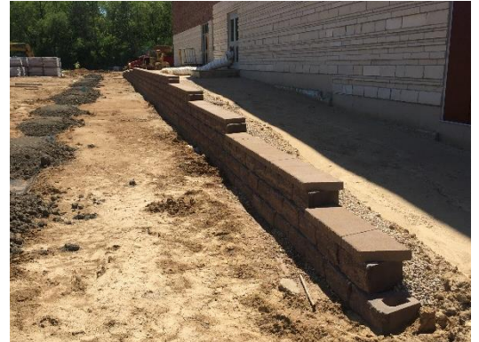
Retaining walls being put in along the Fieldhouse
