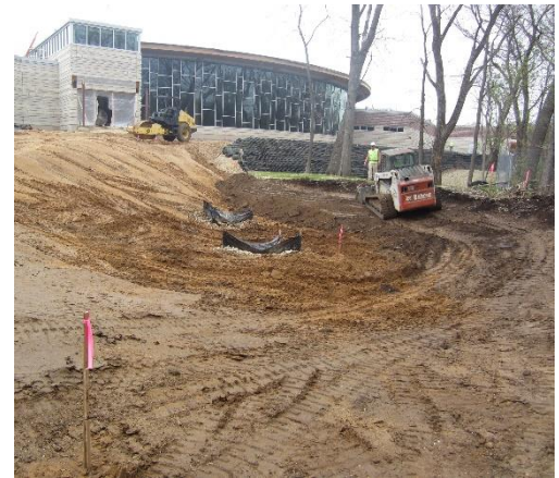
Excavation for the amphitheater has begun - Site
