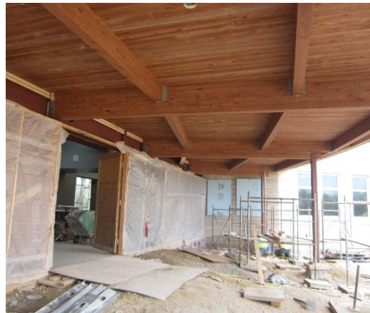
The glu-lam canopy over the main entrance is complete – Area C
