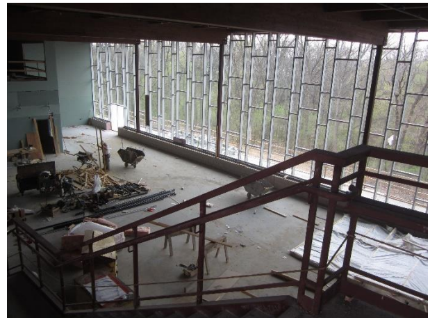
Library Glass has been installed – Area B
