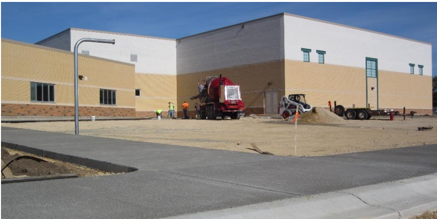
Concrete sidewalks are being poured. The new basketball/playground area is nearly ready for laying asphalt.
