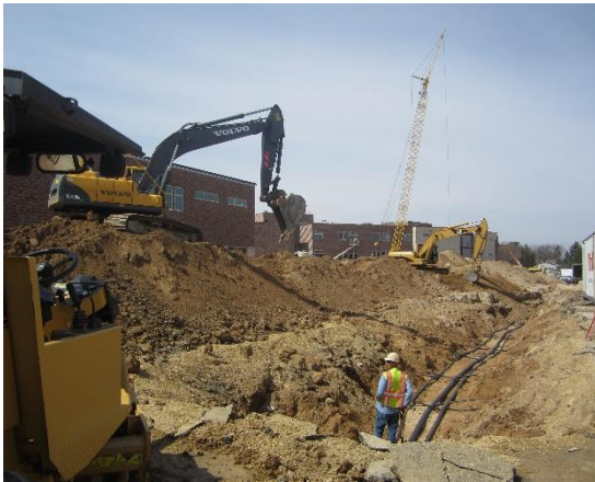
Geothermal trenching and system tie-in is underway
