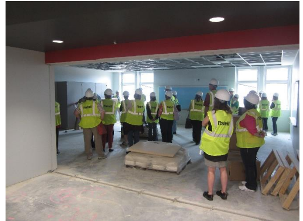
Site tours were provided for the Kromrey staff on Monday 4/21
