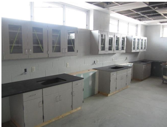
Casework in the 5 th grade classrooms is installed
