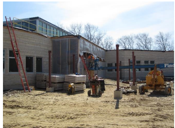
Canopy columns at the main entrance are in place
