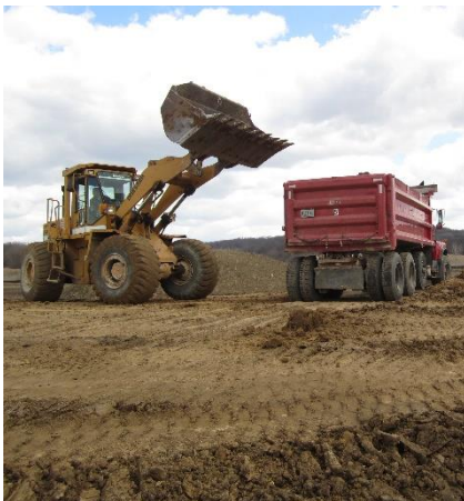
Site Work is Under Way! Material is being removed from the North parking lot to level off this area
