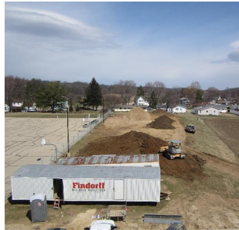
Site Work is Under Way! Material is being removed from the North parking lot to level off this area
