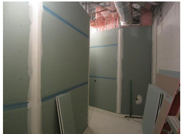
Drywall is up in the new Administration offices - Area C
