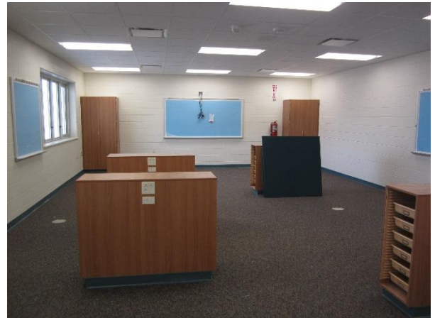
Area D flooring and finishes are nearly complete!
