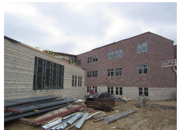
Windows and curtain walls are in place in area C. Area B windows are being installed.
