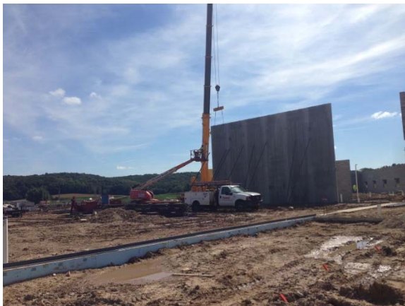
Erect Gym & Fitness Center Pre-Cast – Area F
