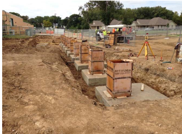
Bus Canopy Foundations
