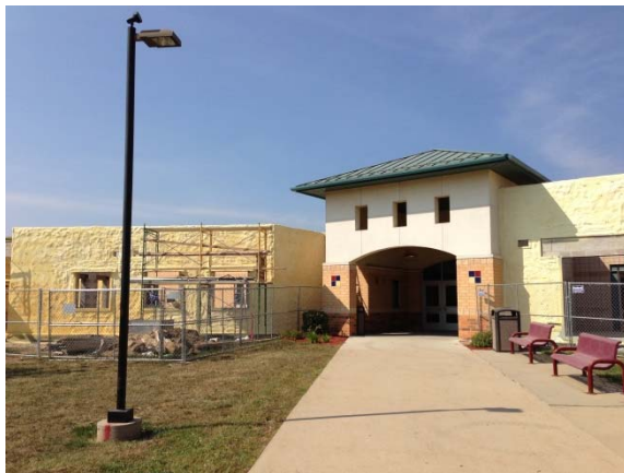
Insulate CMU Walls – Area C (Administration & Commons)
