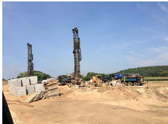
Drill Geothermal Wells
