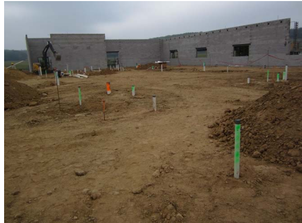
Install CMU Bearing Walls – Area G (5 th Grade Wing)
