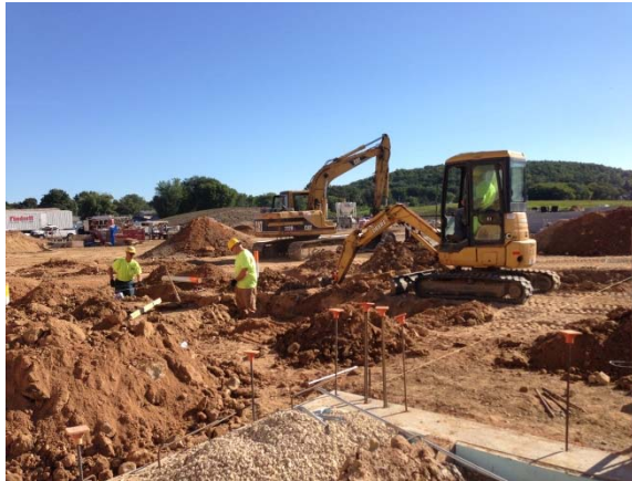
Install Underground Plumbing – Area G (5 th Grade Wing)
