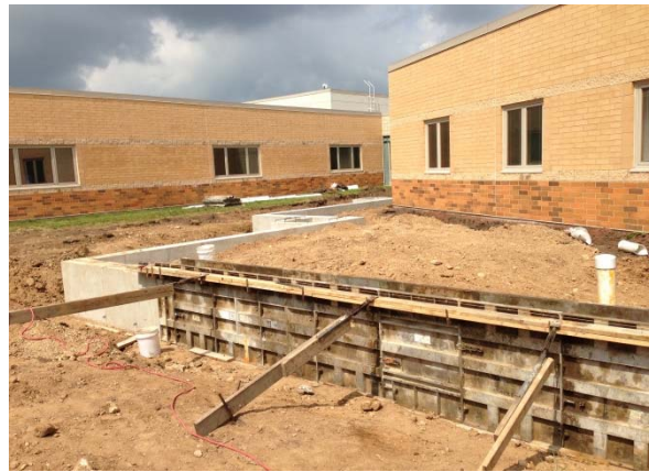
Form and place foundations – Area C (Administration)
