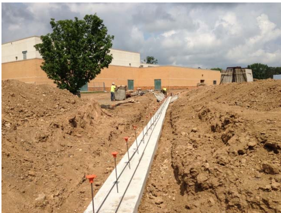
Form and place foundations – Area G (5 th Grade)
