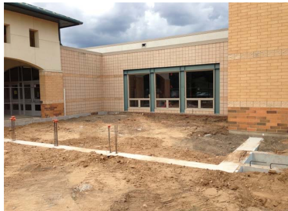
Backfill foundations for start of CMU – Area C (Commons)
