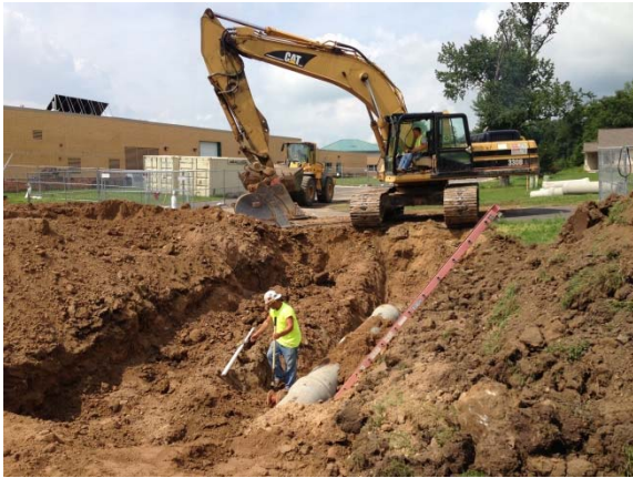
Excavation and installation of site storm drain.
