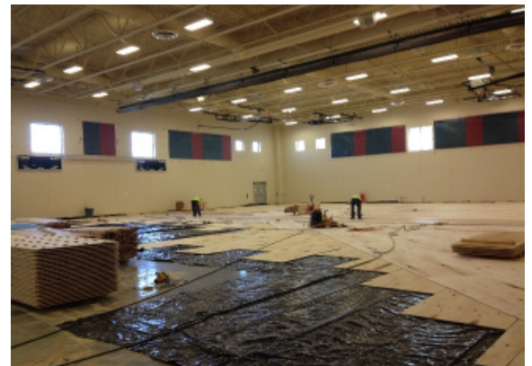
Install Gymnasium Flooring – Area F
