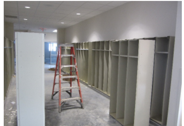
Install Lockers in 5 th Grade Wing – Area G
