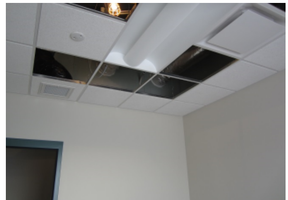
MEPF Trim & Finish in Administration – Area C
