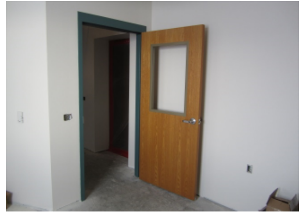
Hang Wood Doors in Administration – Area C
