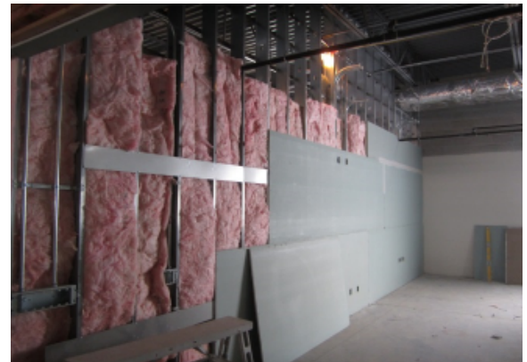
Hang & Finish Drywall in Classrooms – Area G
