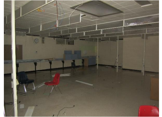
Old building has been vacated – Existing Building
