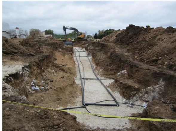
Install Geothermal Circuit – SITE
