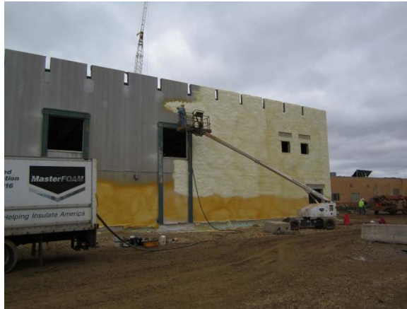
Apply Spray-Foam Insulation – Area F (Gymnasium & Fitness Center)
