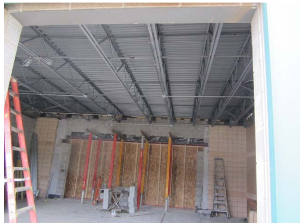
Commons Roof Deck & Wall Demo – Area C (Administration)
