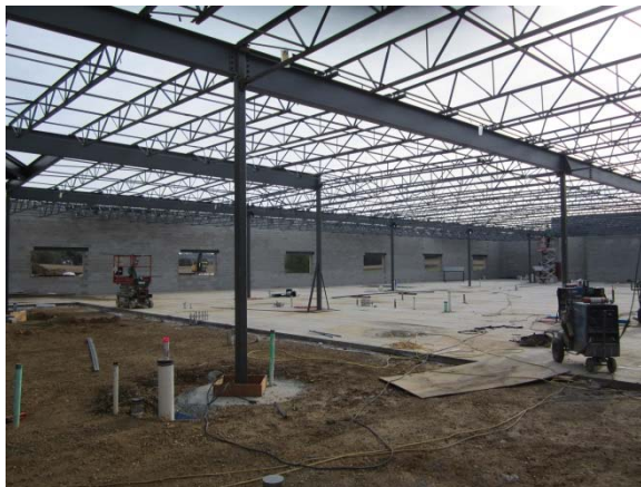
Erect Structural Steel – Area G (5 th Grade Wing)
