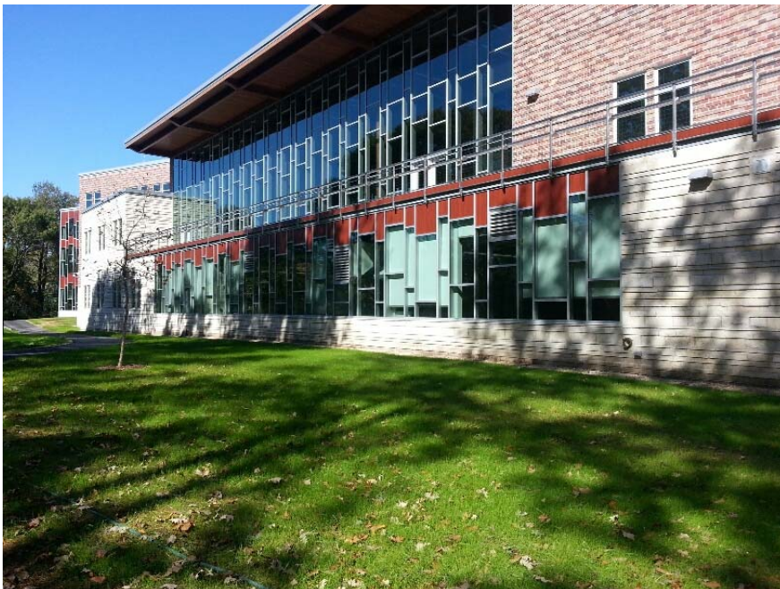
Back side to the three story (Art Rooms & Library) – A & B
