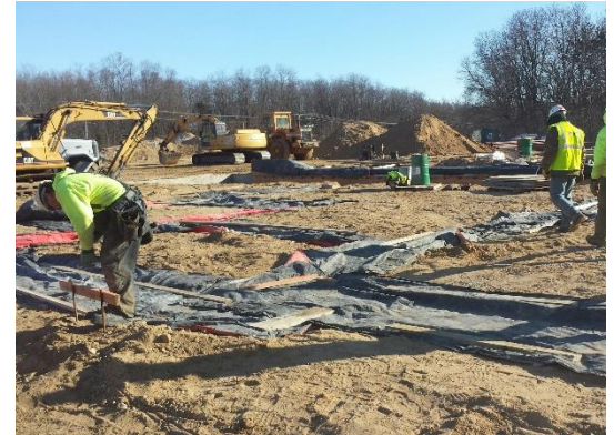
Concrete footings have been blanketed to protect them from the cold weather.
