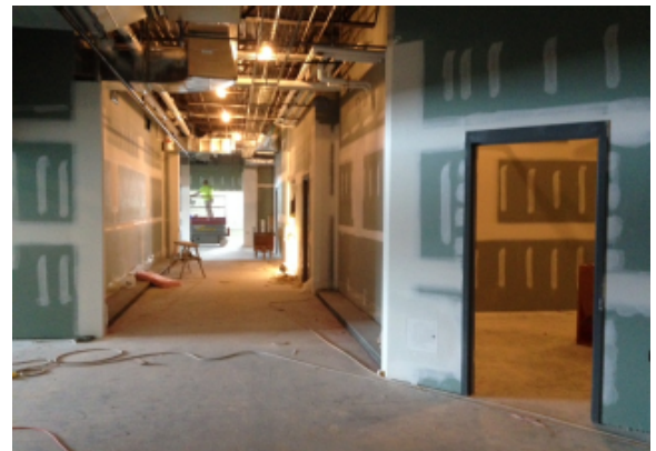
Drywall Finishing – Area G
