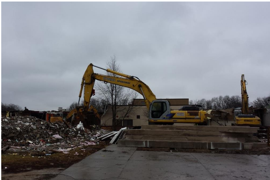
Demolition of the old 8 th grade wing.
