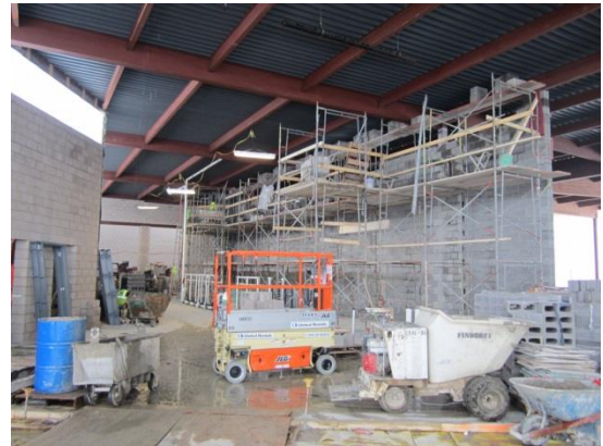
Interior masonry walls have started in the cafeteria.
